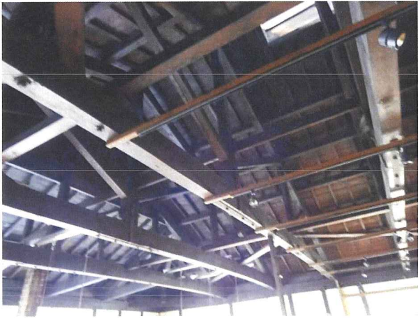
Photo. 2 Full view of King-Post Truss
