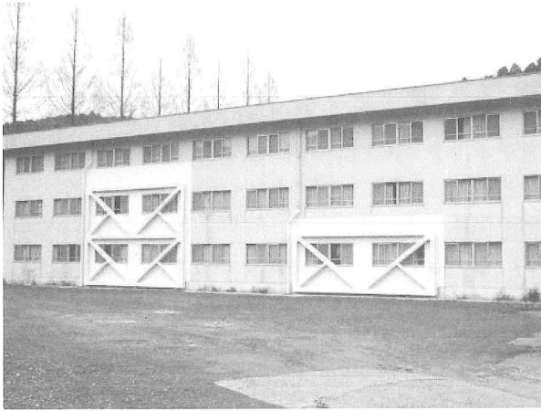
Photo 8 Steel Brace on North Side Wall of Dormitory No.4
